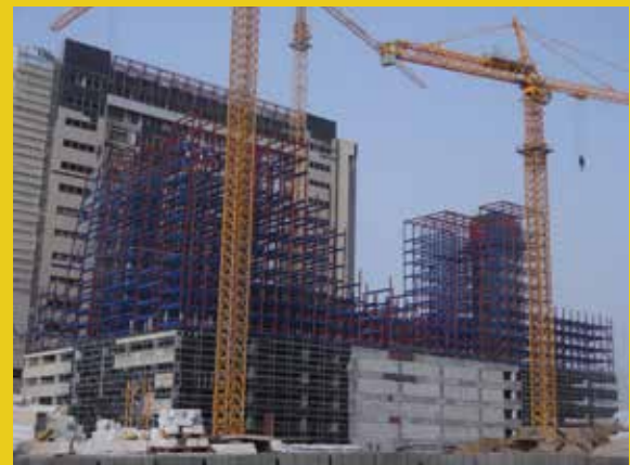
The steel framing is erected. In this development, conventional parking is on the bottom, with the APS above it.
