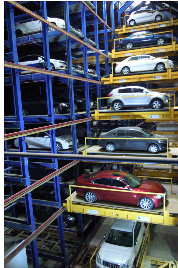
Shown is the interior of the robotic parking garage at the Ibn Battuta Gate Complex.
