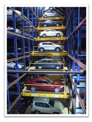
Duplicate electronics and mechanical components and systems ensure that if one machine requires maintenance or repair, a back-up is already operating to keep cars moving into and out of the garage.
